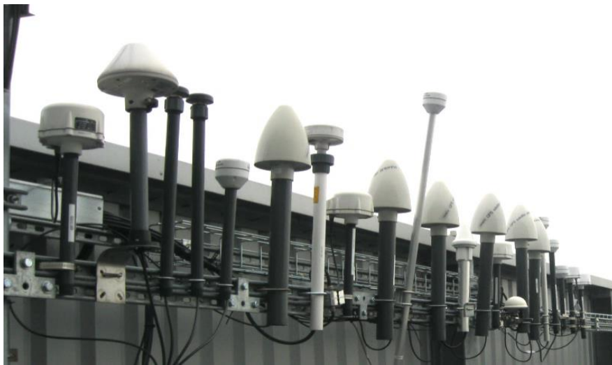
Fig. 16. View of the Roof of an Industrial Plant inside EU. The number of GNSS antennas reflects the typical Industry 3.0, where single PC controls one production line and need one GPS too. The GNSS antennas are placed too close together interfere with each.
